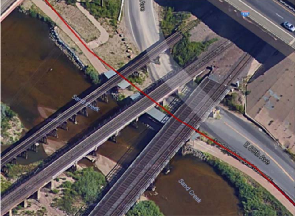
Figure 9: Sand Creek Regional Greenway undercrossing of BNSF and UP trestles; photo courtesy TrailLink.com
