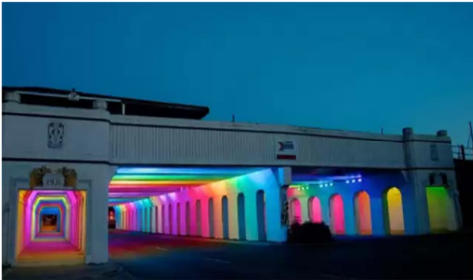
Figure 13: LED lights illuminate the 18 th Street Underpass in Birmingham, Alabama; photo courtesy REV Birmingham, Hal Yaeger and Bill FitzGibbons
