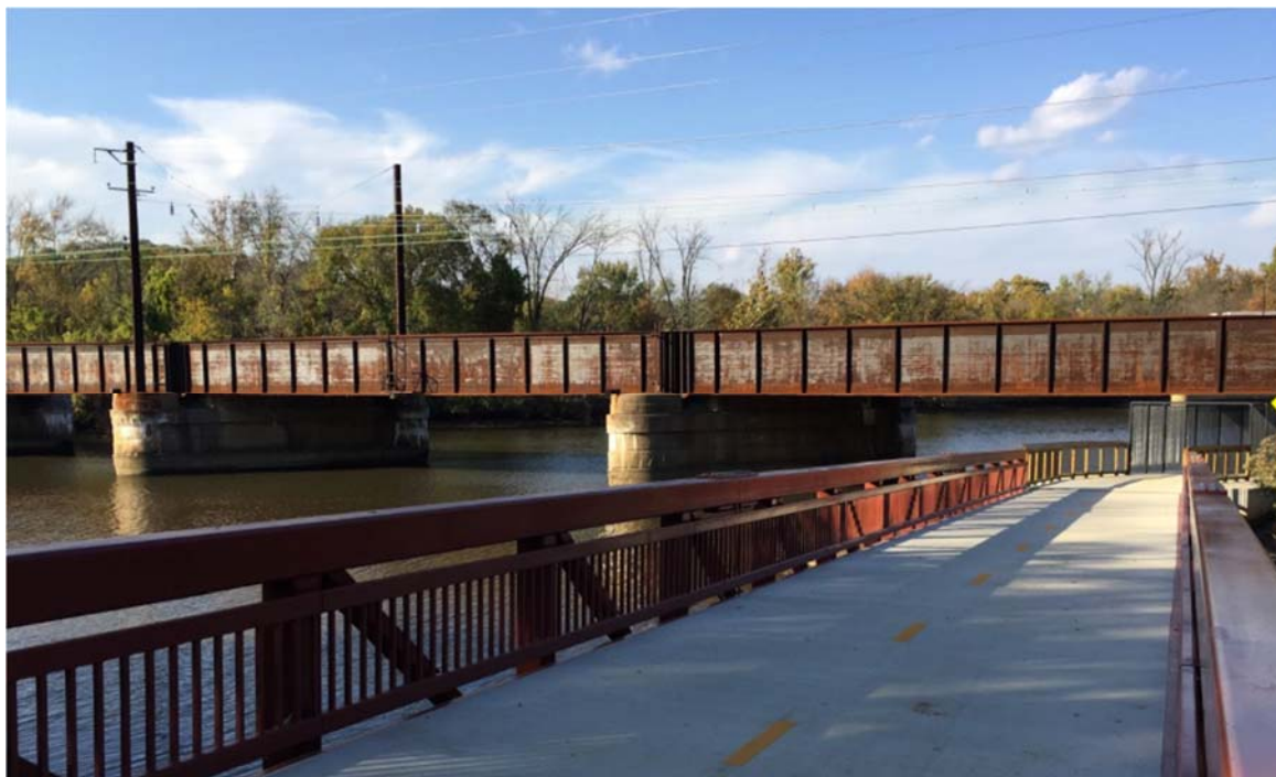
Figure 2: Raised walkway undercrossing of Amtrak's Northeast Corridor line over the Anacostia River along the Anacostia Riverwalk in Washington, D.C.; photo courtesy Greater Greater Washington
