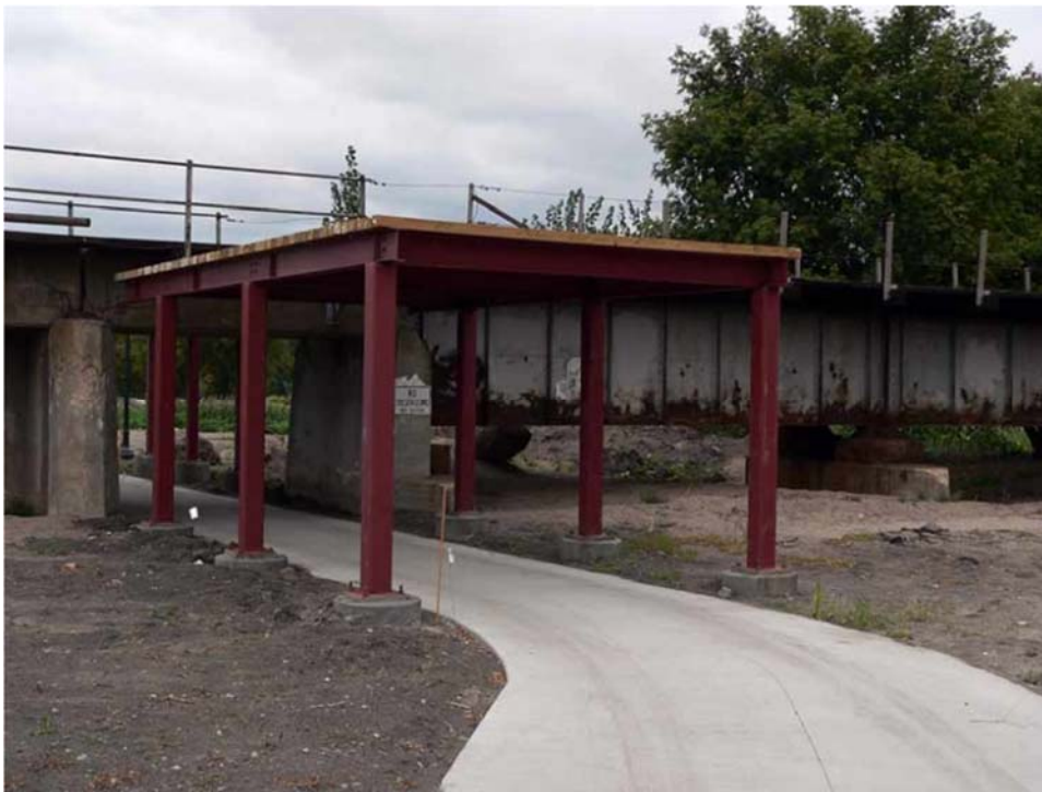
Figure 11: Trail along Red River in Fargo, North Dakota, crossing under BNSF Railway line with metal cover to protect trail users; photo courtesy Stuart Macdonald
