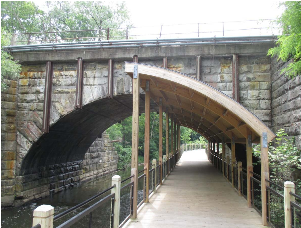
Figure 3: Boardwalk undercrossing of Amtrak line over Mill Creek along the Border-to-Border Trail in Dexter, Michigan; photo courtesy Rails-to-Trails Conservancy
