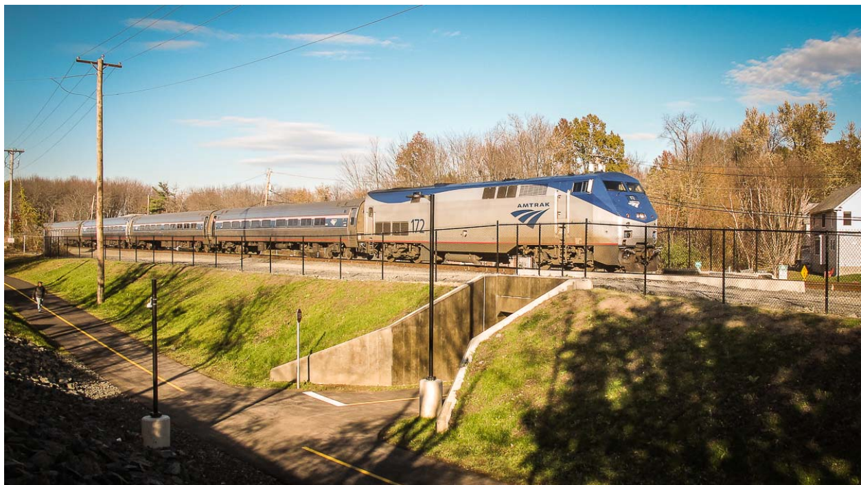
Figure 6: The Northampton Underpass in Northampton, Massachusetts; photo courtesy Trains in the Valley
