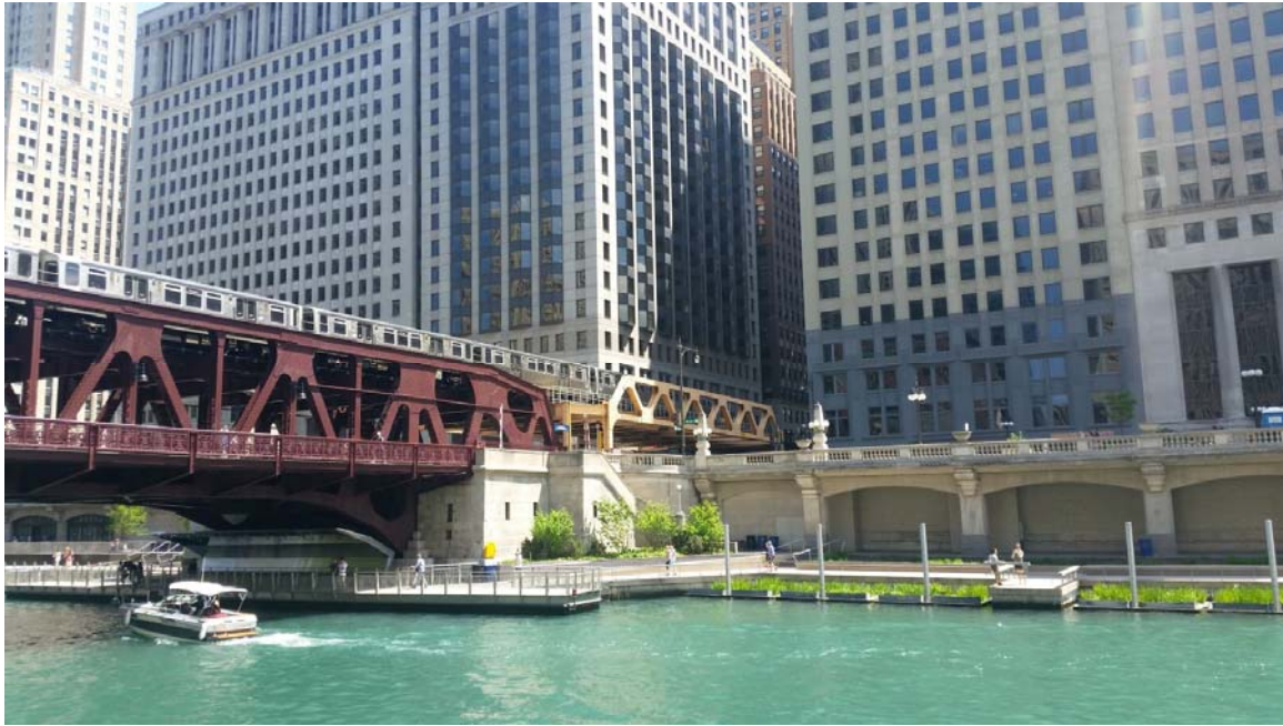
Figure 4: Undercrossing of road bridge along the Chicago Riverwalk in Chicago, Illinois, on new land taken for the project from the Chicago River; photo courtesy Rails-to-Trails Conservancy
